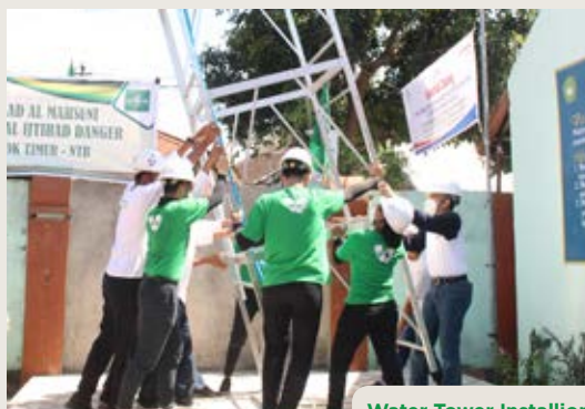
Water Tower Installion
